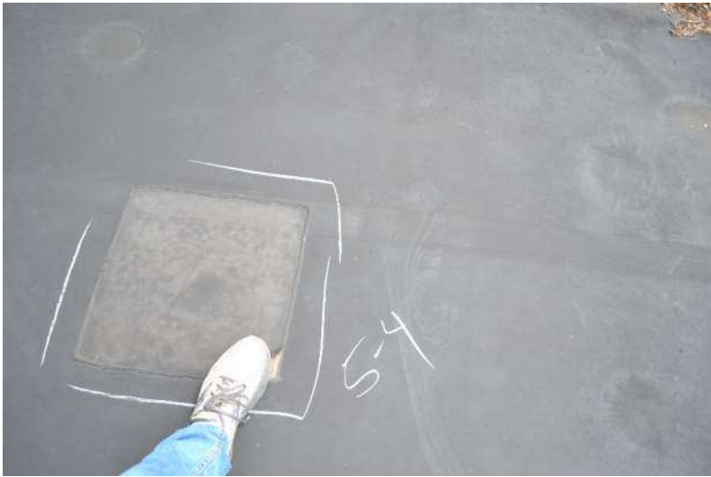
Roof flashings with heat welded edges should be monitored for failure and subsequent replacement/repair.
