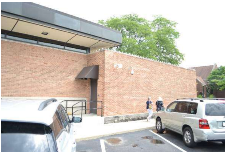
Existing exterior masonry walls.
