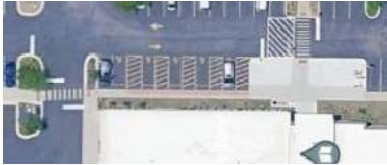
Accessible parking spaces
