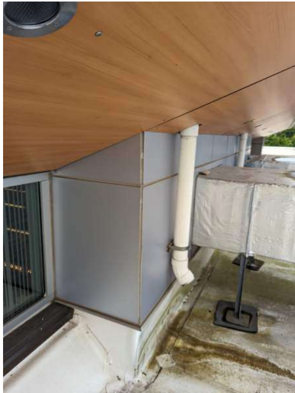
Gutter and downspouts of the skylight atrium portion of the roof.
