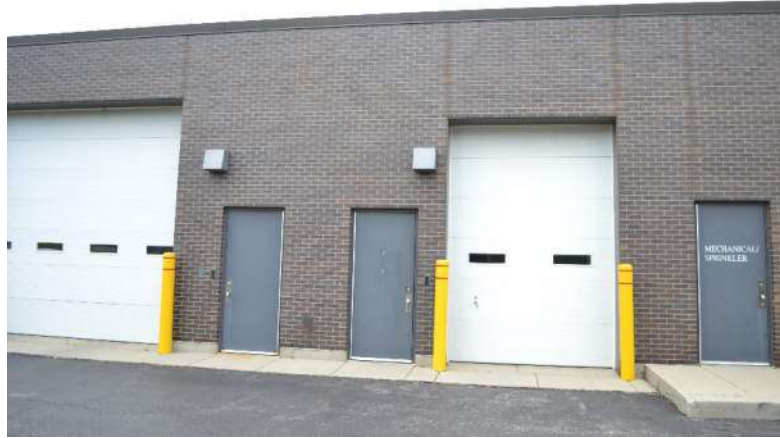
Existing Hollow Metal doors and frames at service door entries/exits.
