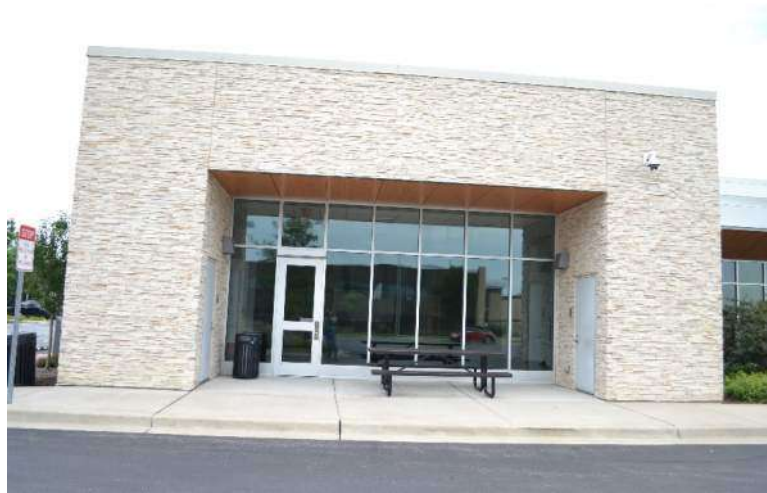
Existing exterior masonry walls.
