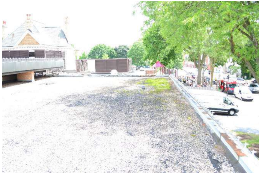
Walkway mats not observed.
