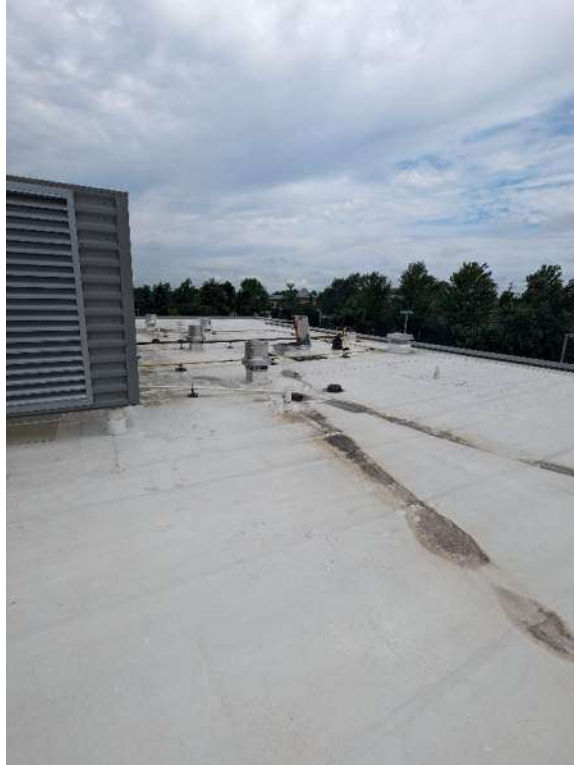
Existing roof surface
