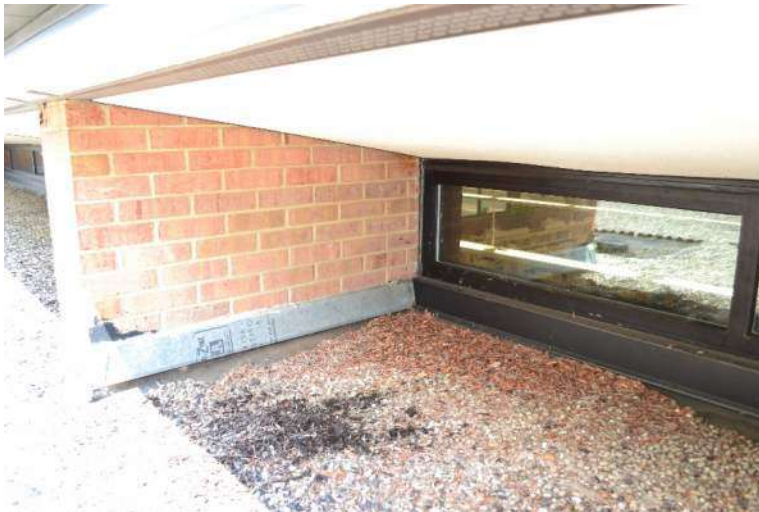
Existing roof surface
