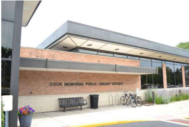
Bike Rack at the main entrance.
